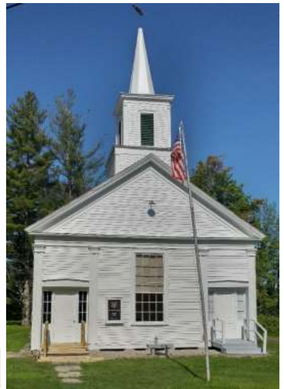
Finished exterior after restoration of steeple, windows and siding
