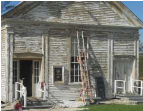
Thorough scraping removed old paint
