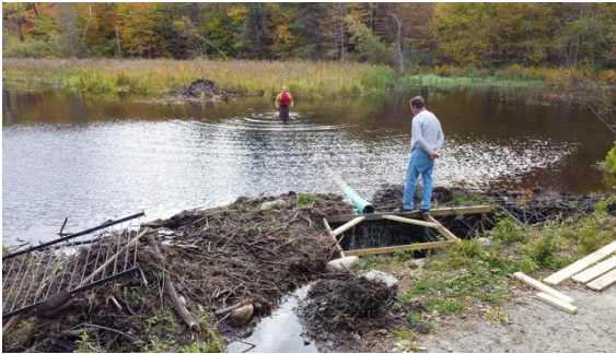
A Beaver Dam Near a Halifax Road Being Outfitted with a Beaver Deceiver © Skip Lisle (photo: David Erickson, Halifax VT)
